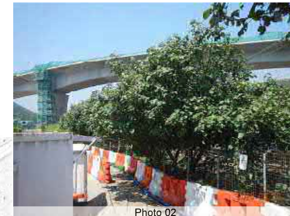
Water barriers with panels for tree protection
