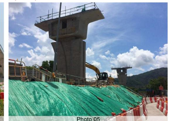
Hydroseeding on soil slopes and sheeting of soil stockpiles to prevent erosion and dust generation with visually unobtrusive material
