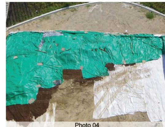
Sheeting of soil stockpiles to prevent erosion and dust generation with visually unobtrusive material
